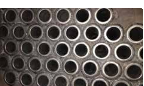
CTI Shield/Seals™ installed in new Waste Heat boiler tubes
