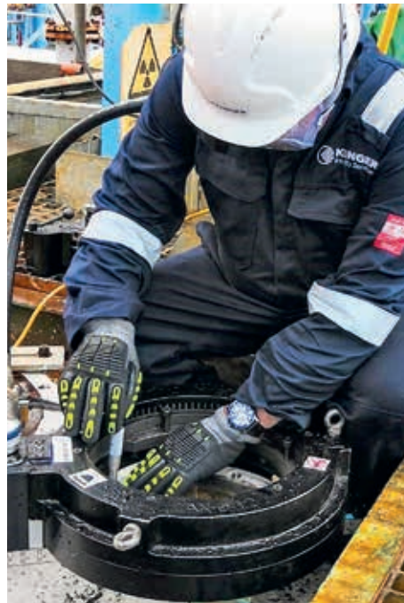
KLINGER Integrity Services employee performing on-site machining repairs
