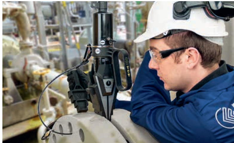
KLINGER Integrity Services employee using a flange spreader
