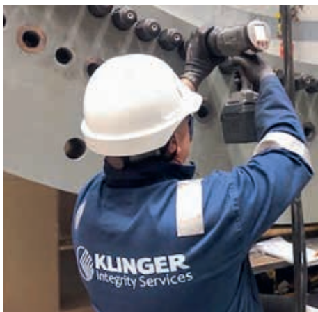
Bolting technician tightening a wind turbine application with state-of-the-art torque equipment
