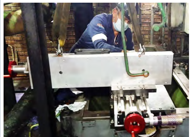
Rigging of Milling Machine into position
